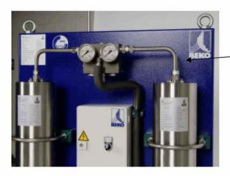
Dismantle the pipe above the adsorption containers.
